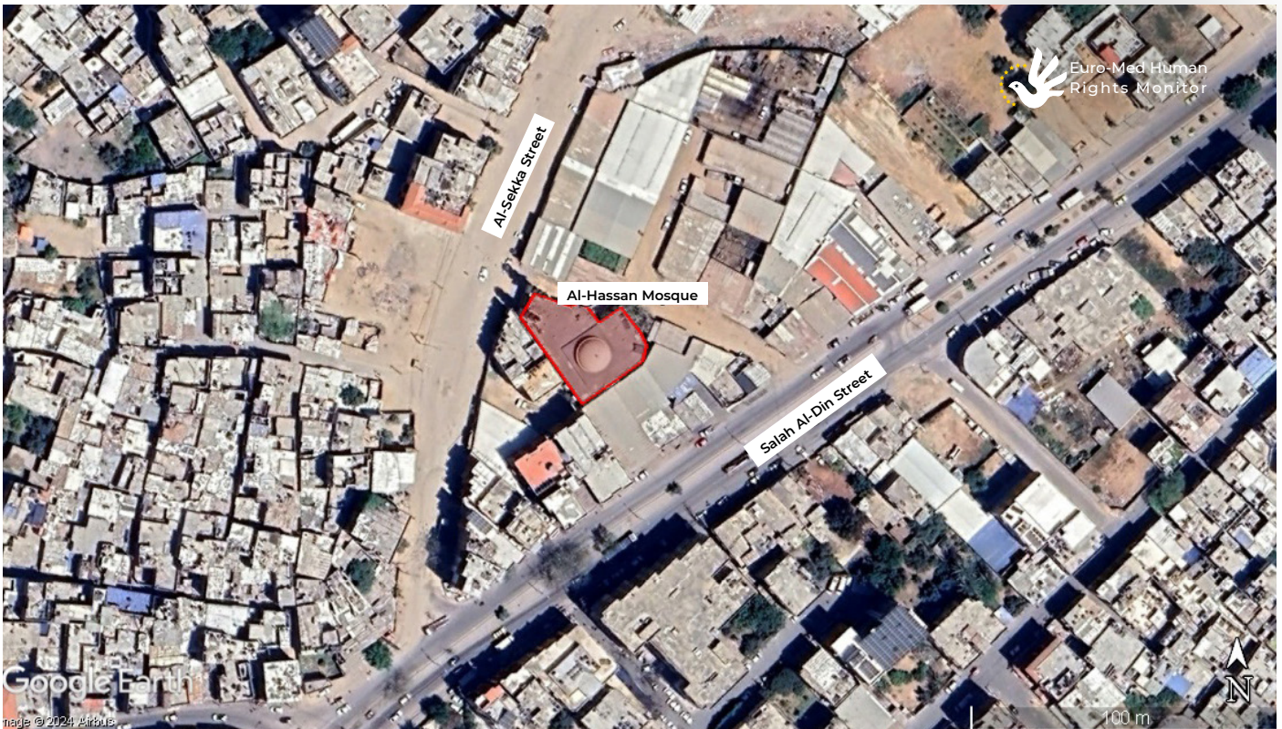
The location of Al-Hasan Mosque near the Sanafor area in Al-Tuffah neighbourhood, eastern Gaza. Image: © 2024 Airbus, Google Earth.
